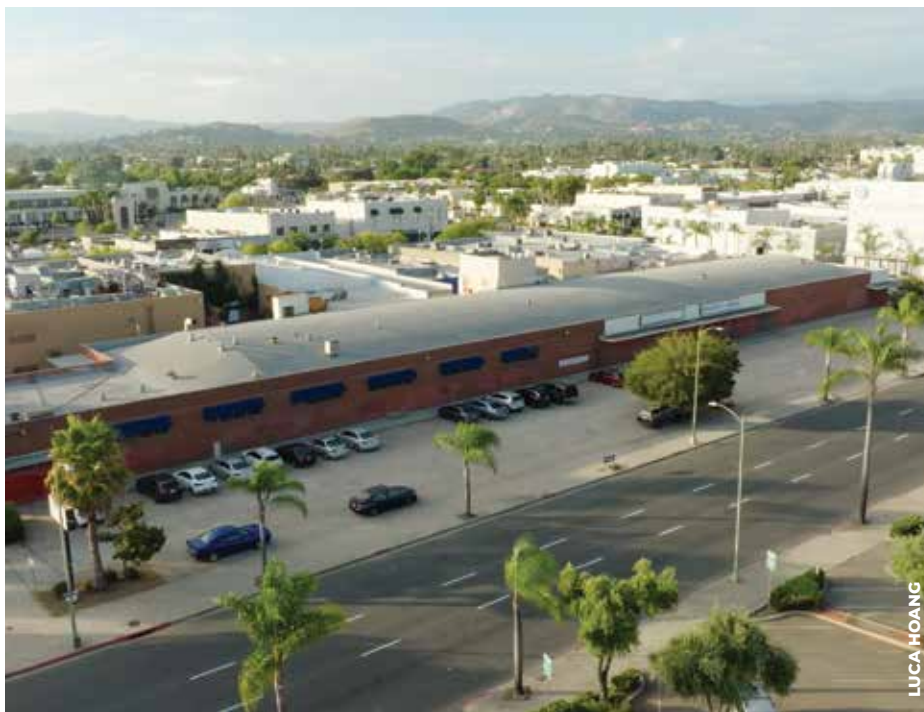
DOUBLING SPACE: The property at 131 S. Broadway in Escondido will be converted into a new Creative Arts Academic Complex for John Paul the Great Catholic University.
