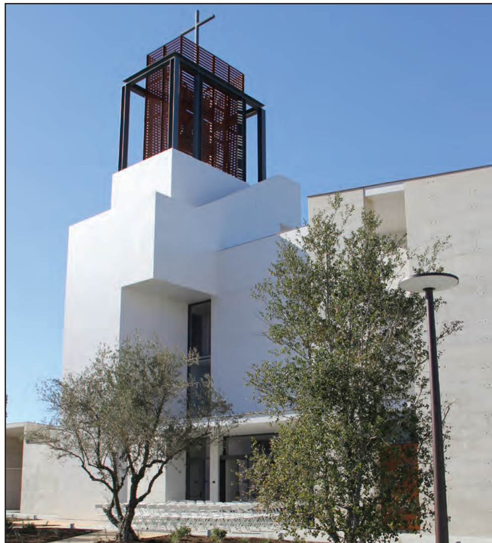
NEW CHURCH: A wooden "Tower of Light" tops the newly dedicated St. Thomas More Church in Oceanside.
